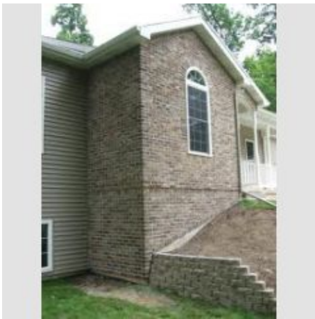
Thin Brick used as an accent on exterior siding.
